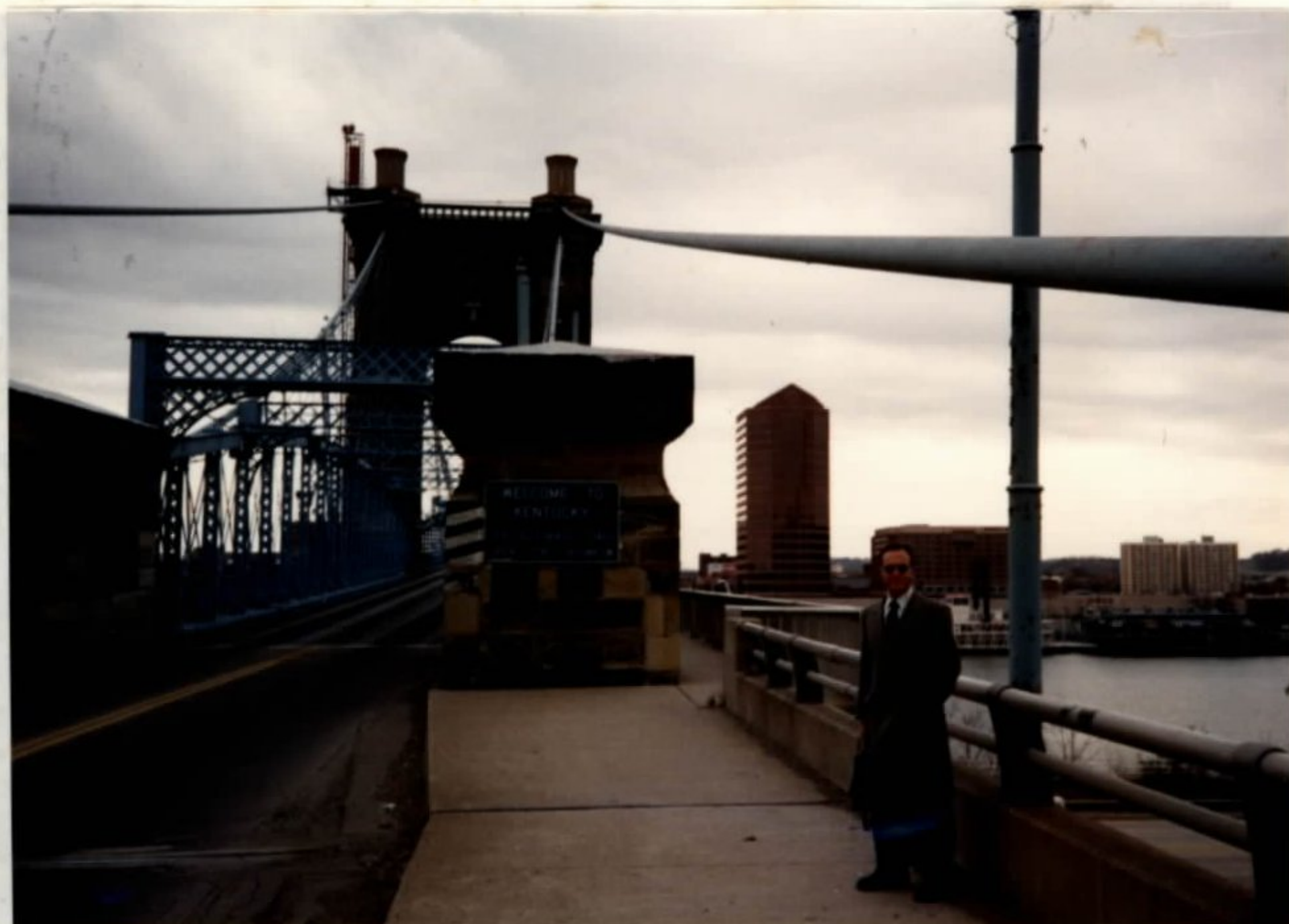
AUTOMATIC STATION ON OHIO RIVER - CINCINNATI -
