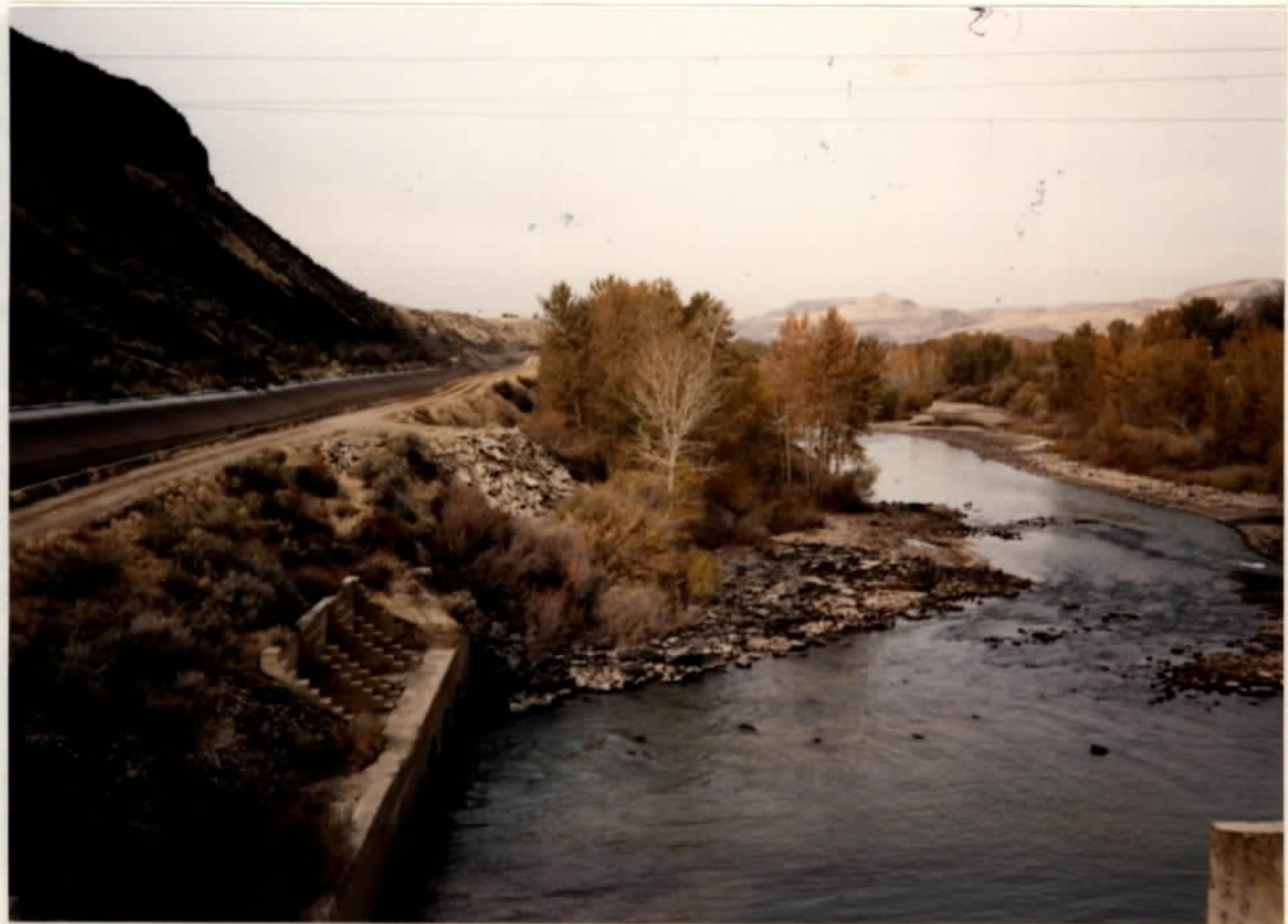
BOISE RIVER DOWNSTREAM DIVERSION DAM STATION (CLOSE TO BOISE)
