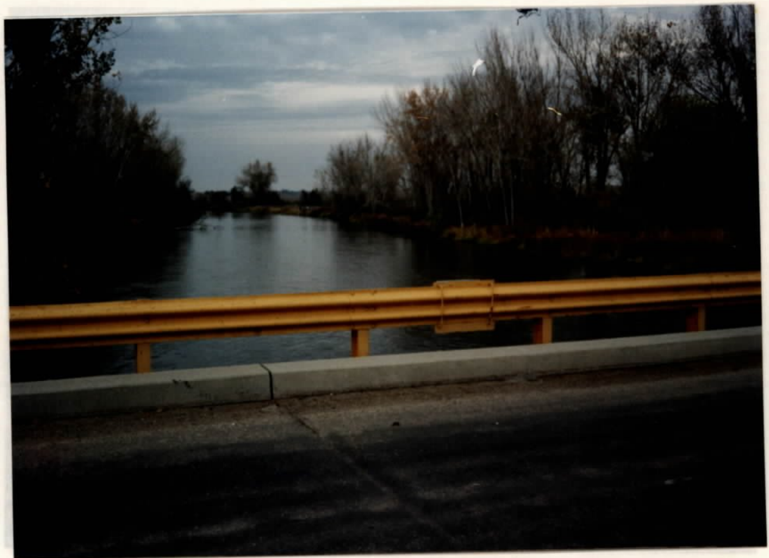
BOISE RIVER AT BOISE AUTOMATIC STATION
